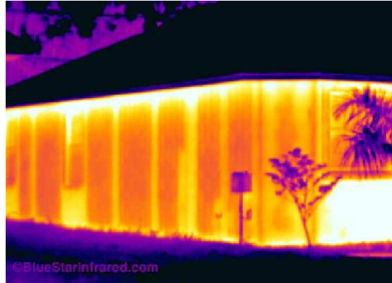
Thermal image highlighting energy loss typical of standard CBS type construction.
